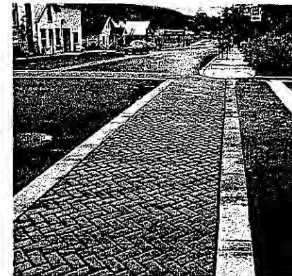
Not Appropriate: Simulated brick or stone from stamped and tinted concrete
