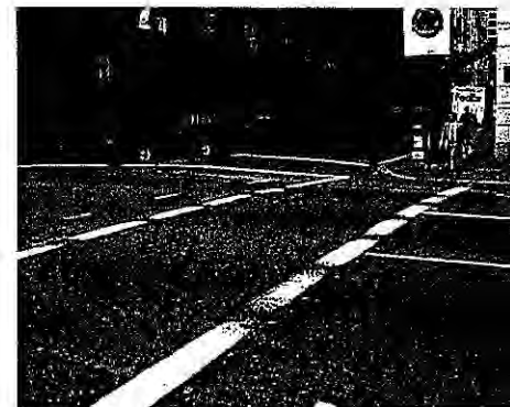
Not Appropriate: Single stripes wear out in heavy traffic and only minimally define the pedestrian zone
