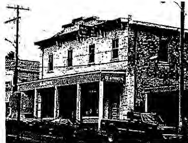
Appropriate: Two-story brick building
