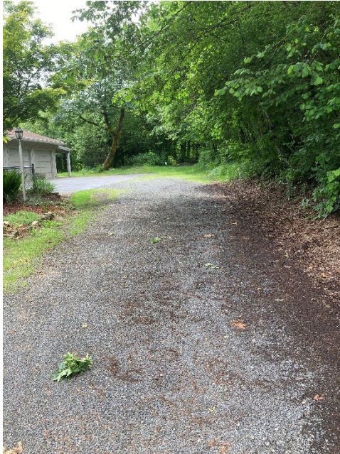
Above – Del Rey (east) looking west
