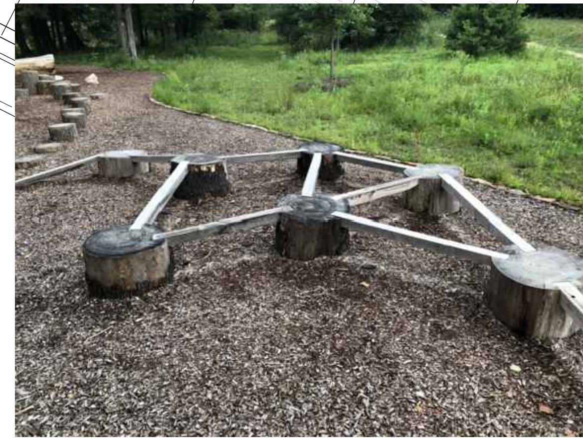
2 STUMP OR BURIED LOG ENDS WITH BEAM BALANCE TIMBER NOTCH INTO STUMP/LOG ENDS
