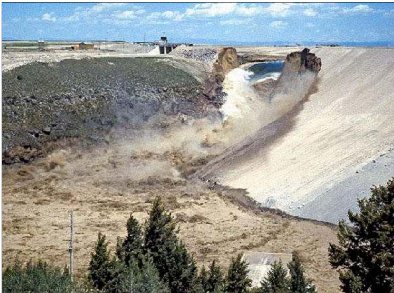
Figure 10-1. Teton Dam Failure, 1976
