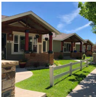
1-story, attached, single-family 4 to 8 units
