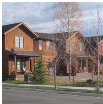
2-story, attached, single-family townhomes
