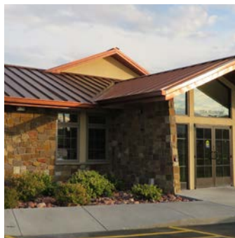
Stone siding with metal roof
