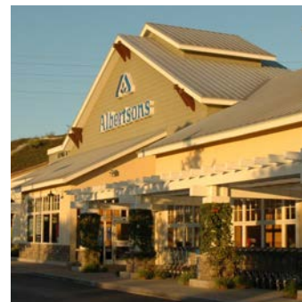
Stucco mix with pitched roofs
