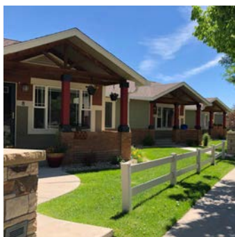
1-story, attached, single-family 4 to 8 units
