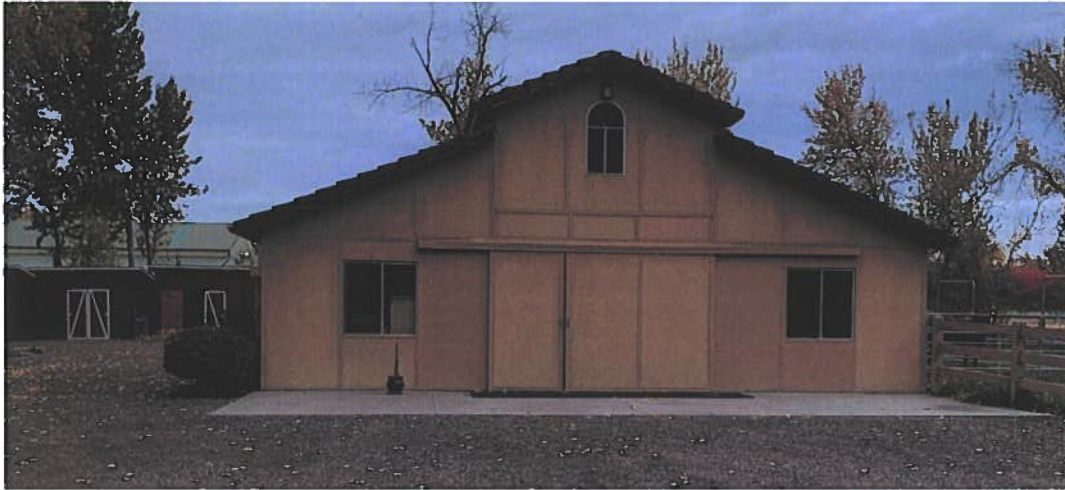
South face of existing barn.
