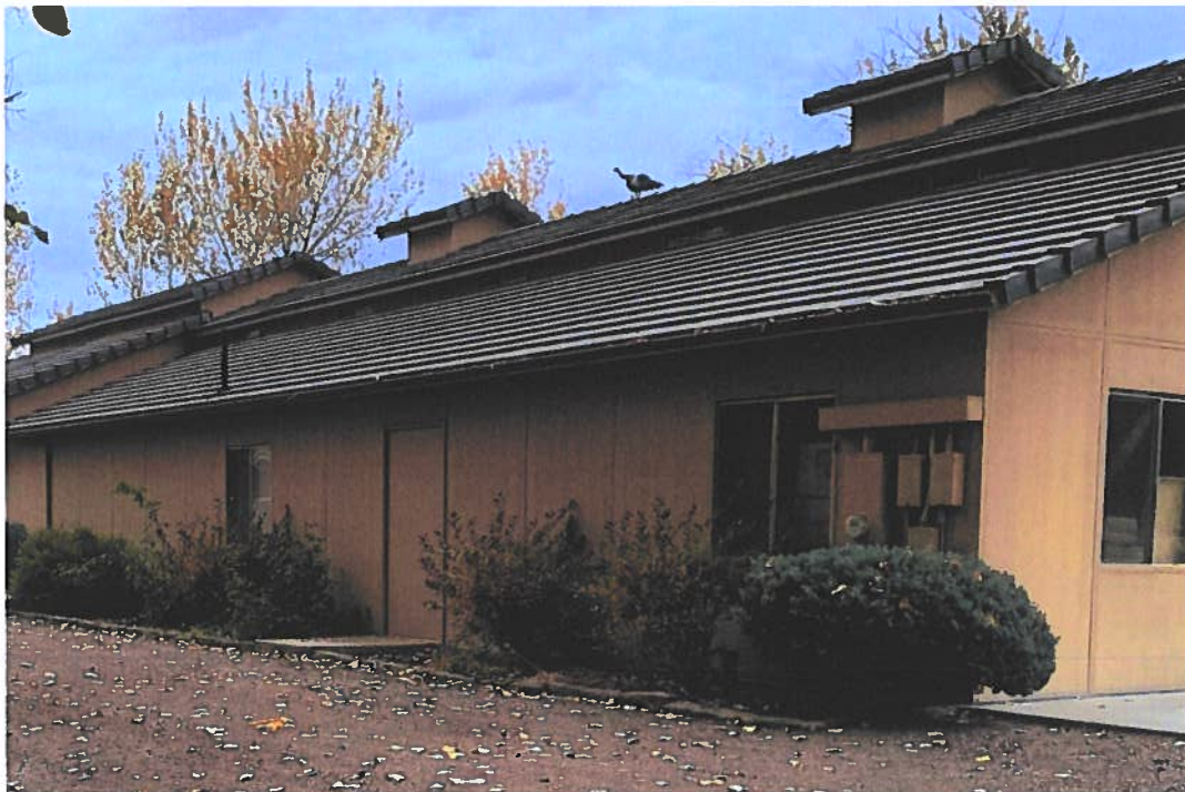
Southwest corner of existing barn.
