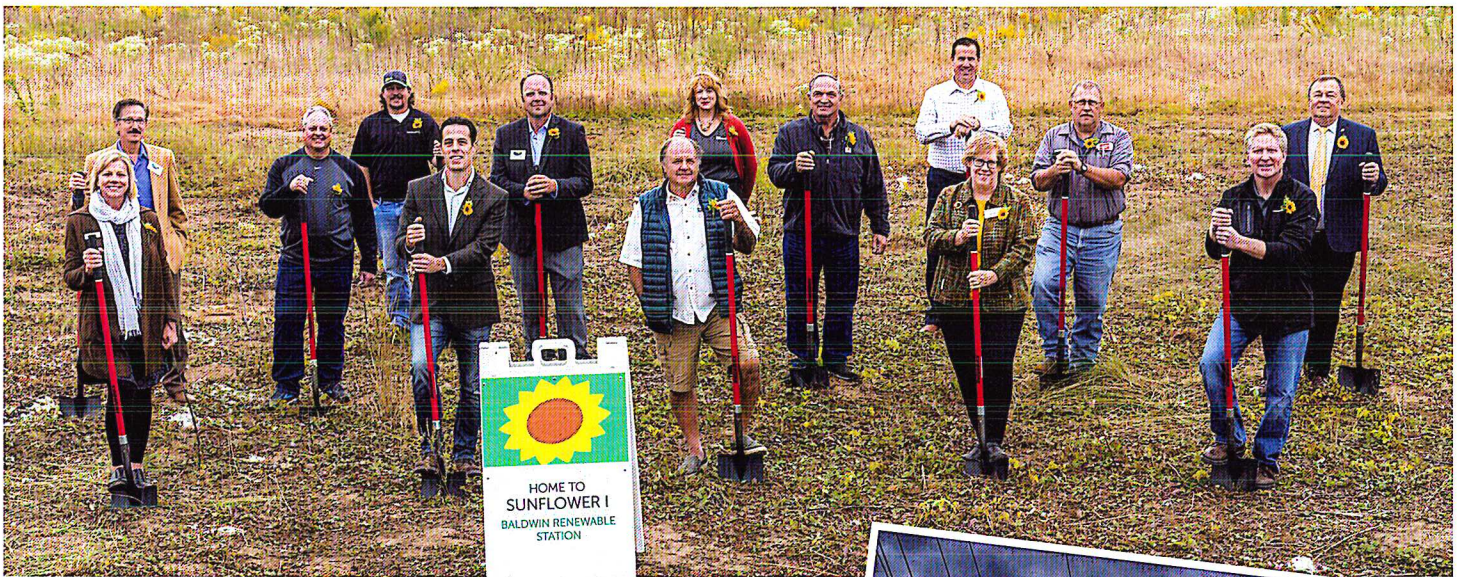
A groundbreaking event was held this fall for Sunflower I. Our newest solar array located near Princeton will produce 5,400 MWh of annual energy, which is equivalent to the usage of 530 homes.
