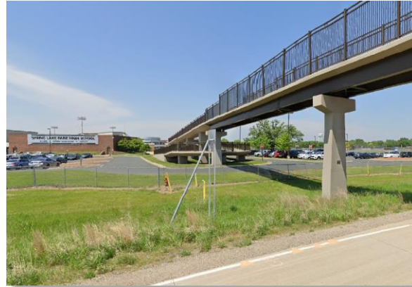
Pedestrian Bridge at S.L.P. High School
