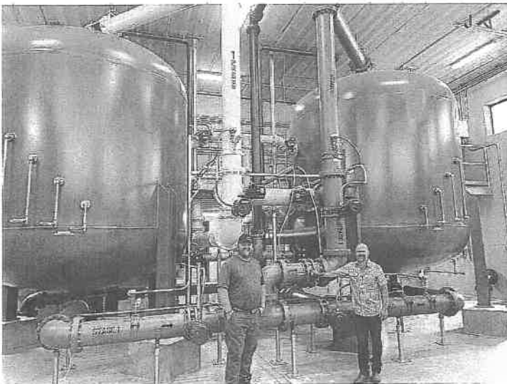
Jon Stueve and Ryan Capelle in front of the filters with the granular activated carbon.
