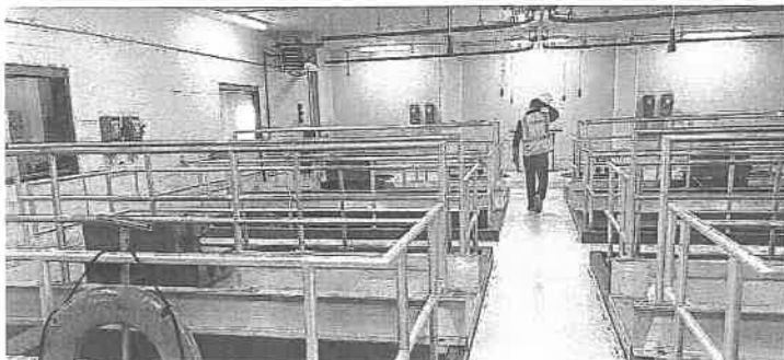
The flocculation basins and filters in Two Harbors.
