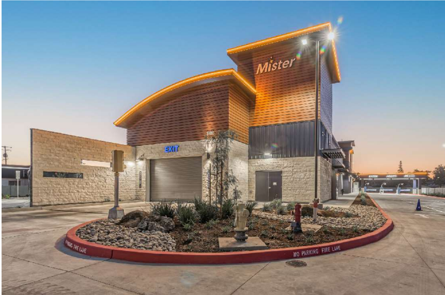
EXHIBIT 9 PHOTO OF SIMILAR WALLS AT EXISTING SITE
