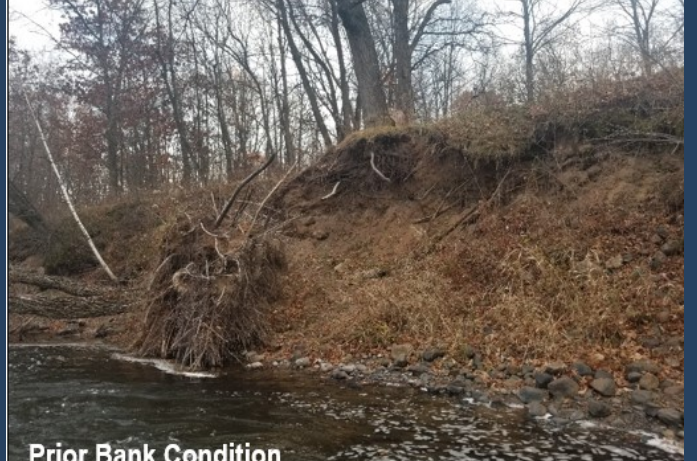
Prior Bank Condition
