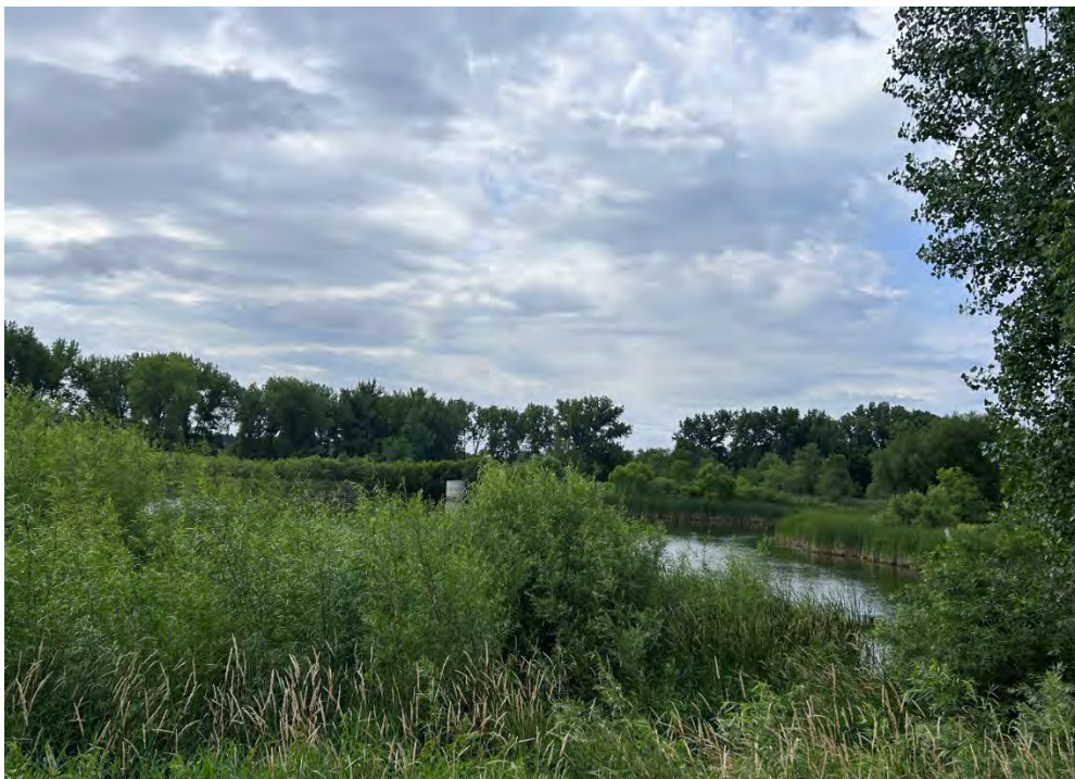
Figure 9 Shoreview Rice Fields Stormwater Reuse Pond at 5880 Rice Creek Pkwy, Shoreview, MN 55126
