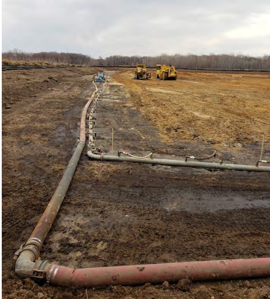
Figure 12 Construction Dewatering Site
