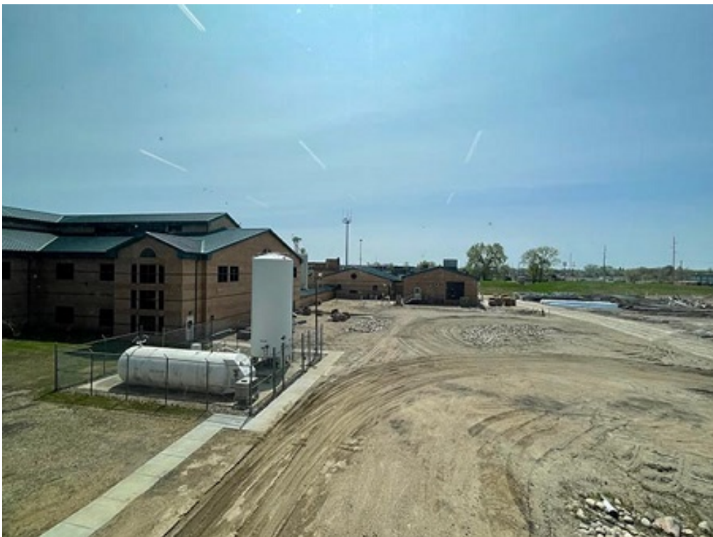
The existing plant is to the south of the new dewatering building.
