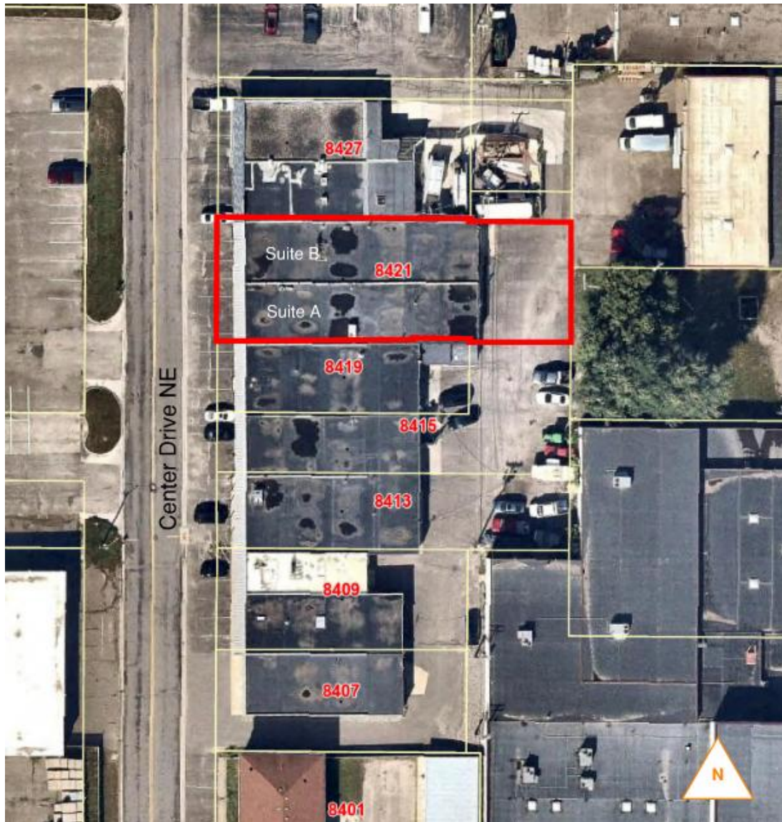
Figure 1: Aerial of the site, per Anoka County GIS. Parcel lines are shown in yellow. Subject property is outlined in red, with the suites/units labeled.
