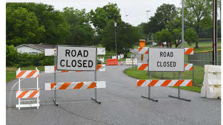
MAINTENANCE OF TRAFFIC IS KEY TO SAFETY
