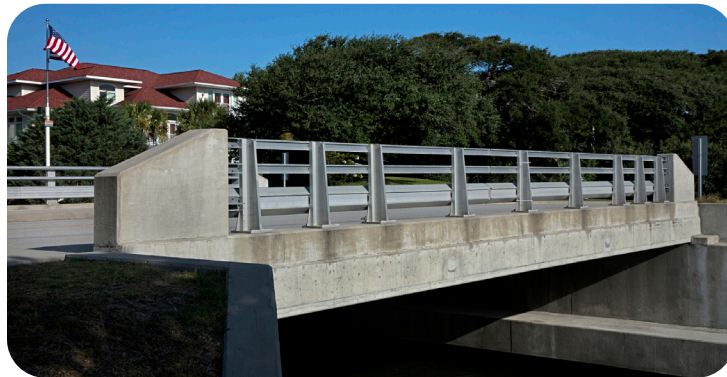
Mimosa Boulevard Bridge in Pine Knoll Shores
