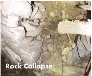
Tunnel Collapse
