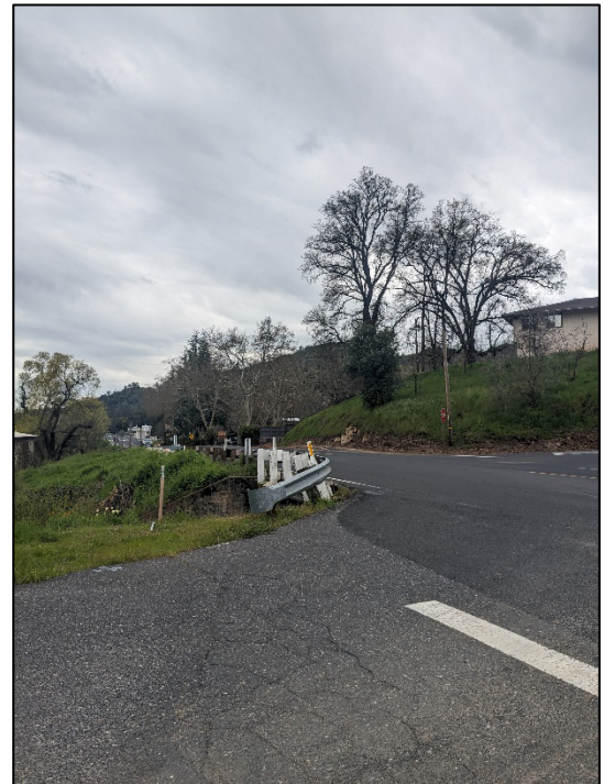
Southgate Drive and SR 49
