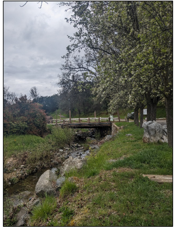
Southgate Drive Bridge Over Sonora Creek
