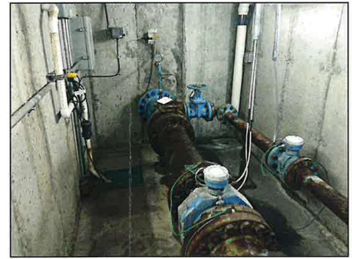
EXISTING PIPE CONDITION IN VAULT
