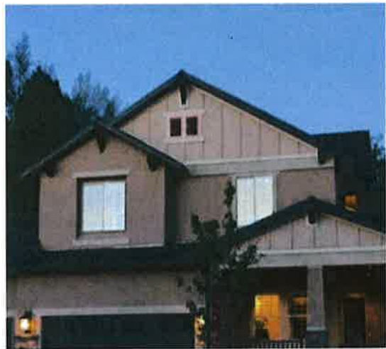
Complex roof lines, exposed beams and covered porch.
