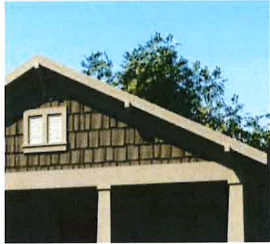
Exposed beams and shingle siding.
