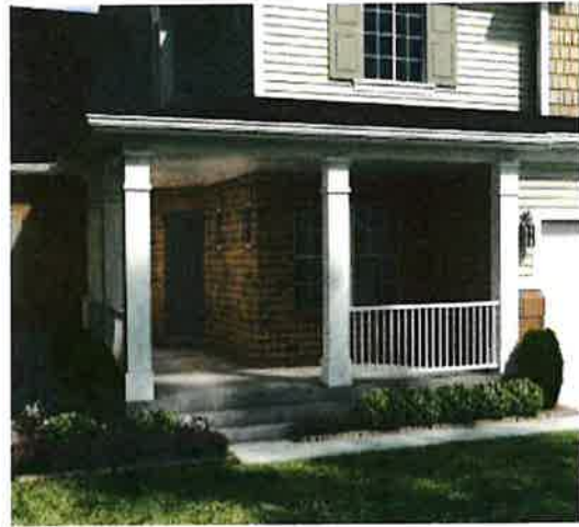
Wrap-around porch with wood handrails.
