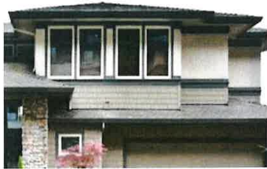
Low pitched roof, broad overhangs, material lines that reinforce horizontal.
