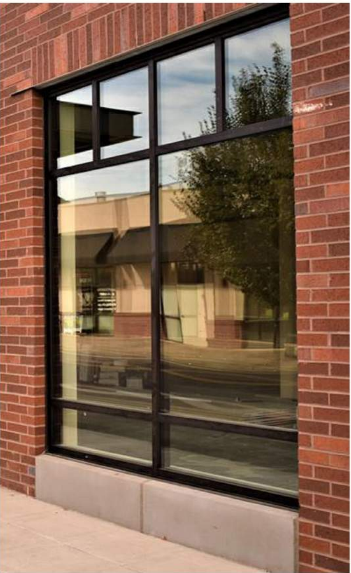
ALUMINUM FRAMED STOREFRONT & WINDOWS BASIS OF DESIGN: KAWNEER PRODUCT & COLOR: TRIFAB 450 FRAMING SYSTEM, BLACK
