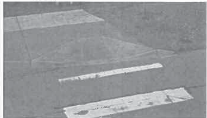
EXISTING RAMP PHOTO
