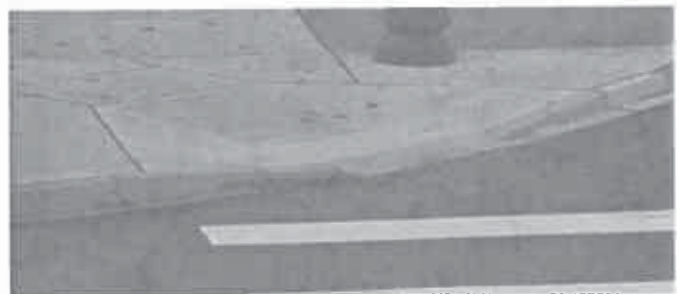
EXISTING RAMP PHOTO
