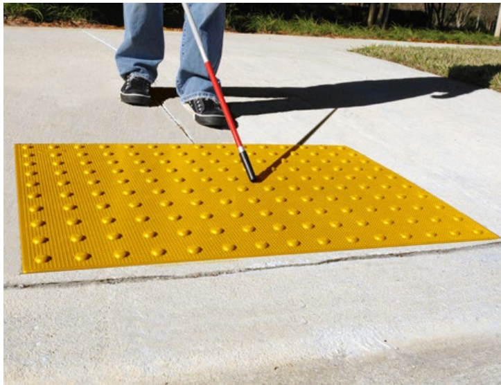
Compliant Truncated Domes
