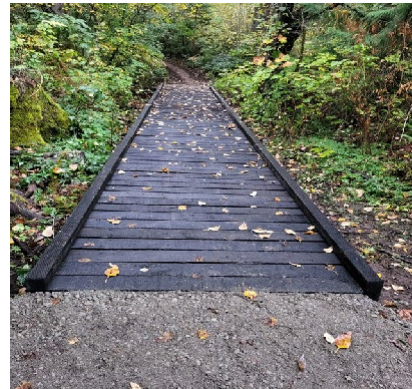
Steller Boardwalk Replaced
