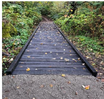
Steller Boardwalk Replaced
