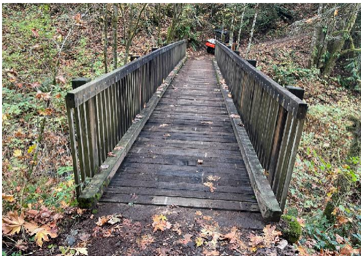
Deep Creek Bridge Deck Partially (left) and Fully (above) Replaced
