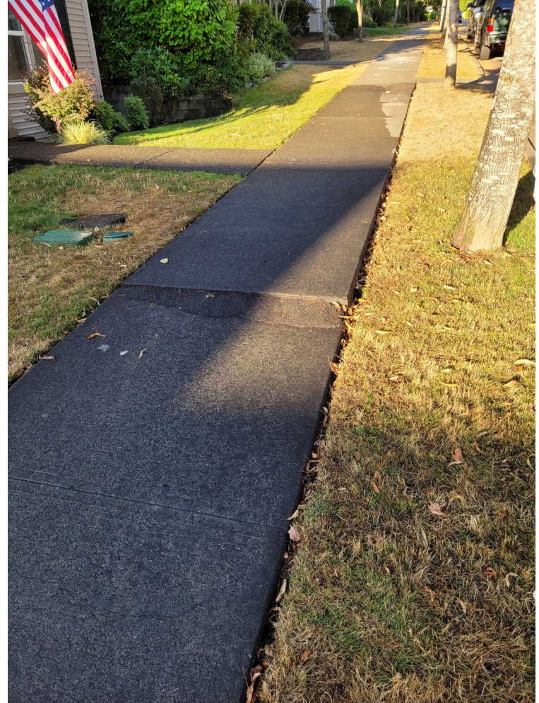
Cold Mix Asphalt
