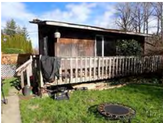
12. Looking northeast at shed
