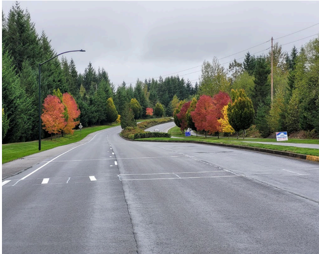
Snoqualmie Parkway Restoration
