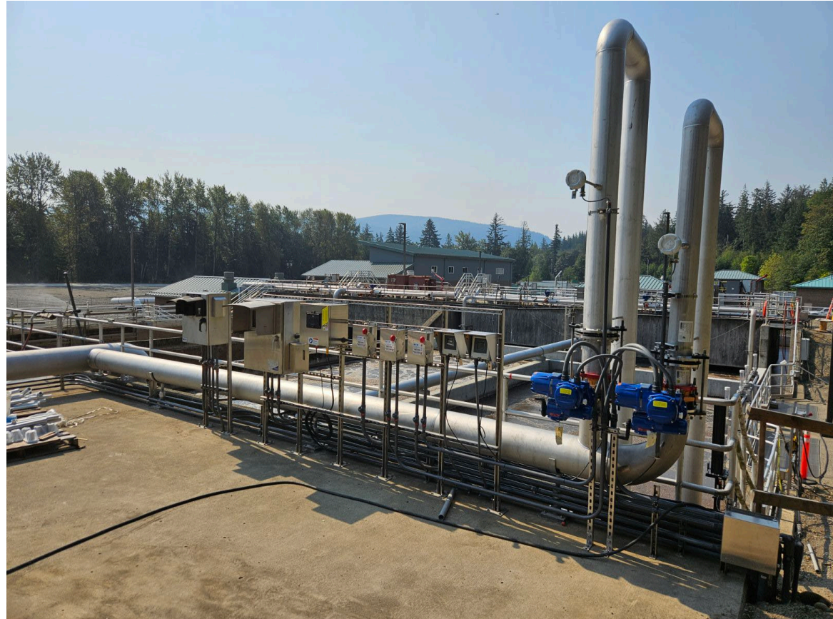
WRF 3 – In progress
