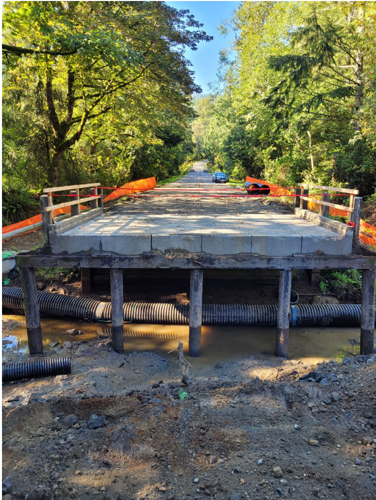
Kimball Creek Bridge Replacements – In Progress
