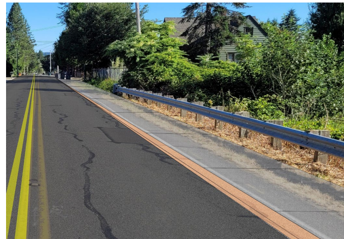
384 th Sewer Main/Sidewalk
