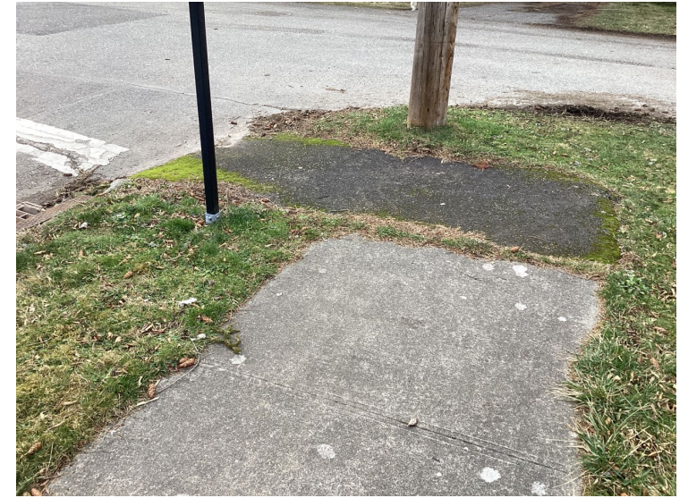
No Detectable Warning Surface
