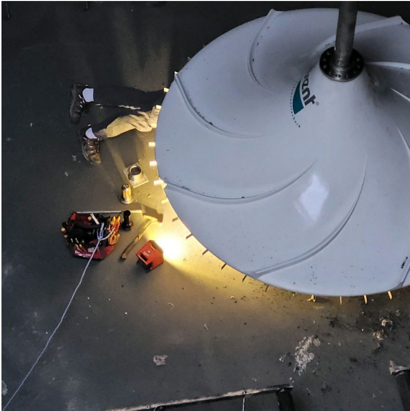
Repairing a digester at the Wastewater Plant
