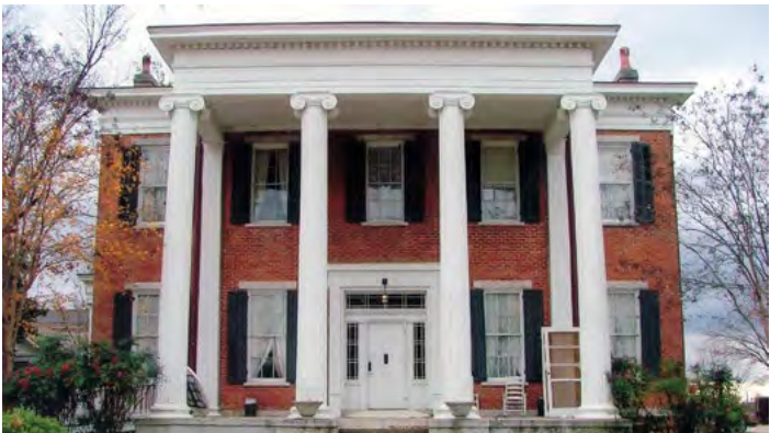
[44] Not Recommended: (a-b) The historic character of this plantation house (marked in blue on plan on opposite page) and its site was diminished and adversely impacted when multiple new buildings like this (#3 on plan) were constructed on the property (c).
