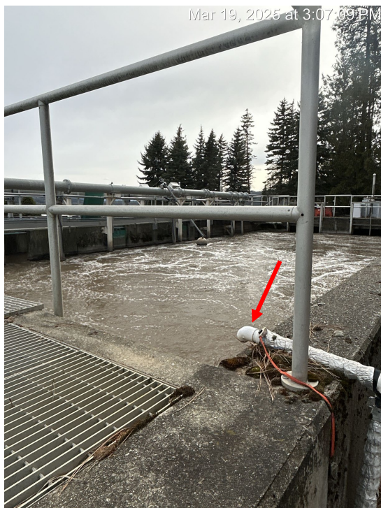
Photograph 5. Aeration basin overview with groundwater pipe discharging to the basin indicated with red arrow, facing southwest.
