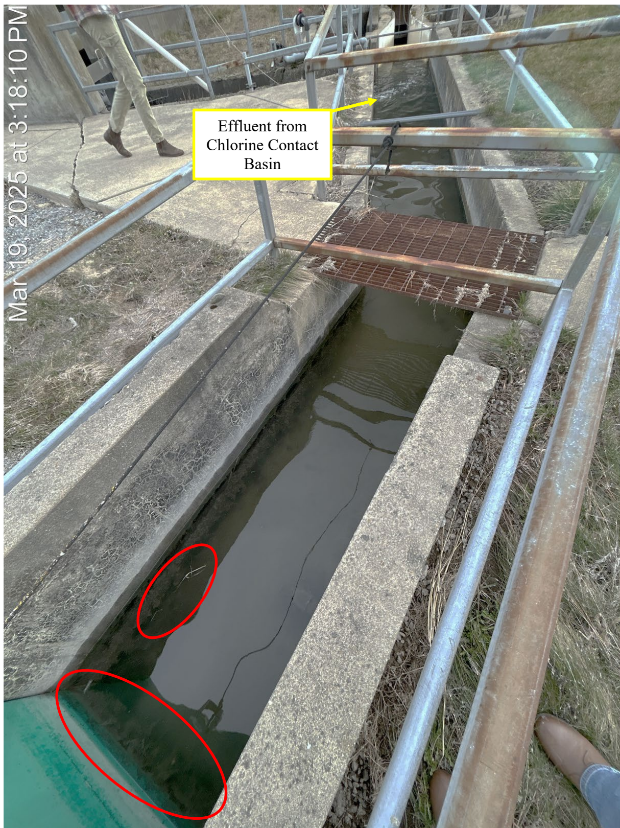
Photograph 10. Upstream of chlorine contact chamber effluent to receiving waters, algae and debris indicated by red circles, facing southeast.
