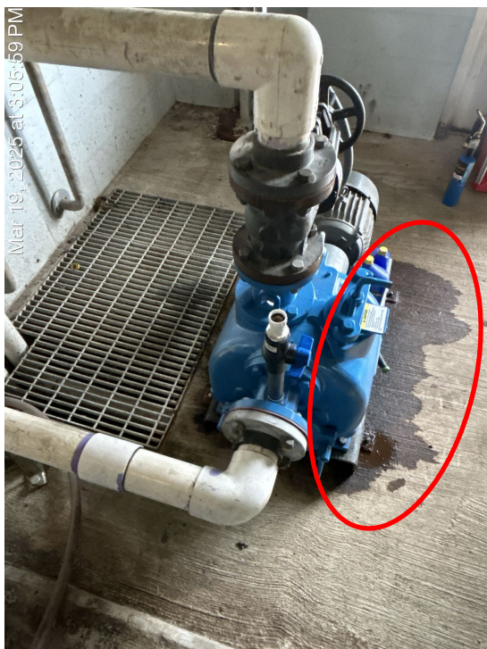
Photograph 11. Breezeway pumping building, oil bordering northern pump indicated by a red circle.
