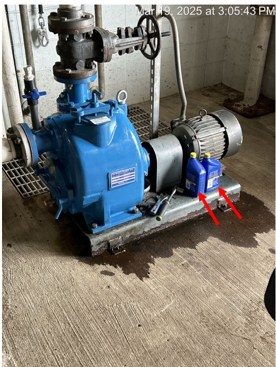
Photograph 12. Breezeway pumping building, northern pump leaking oil, containers without secondary containment indicated by red arrows.
