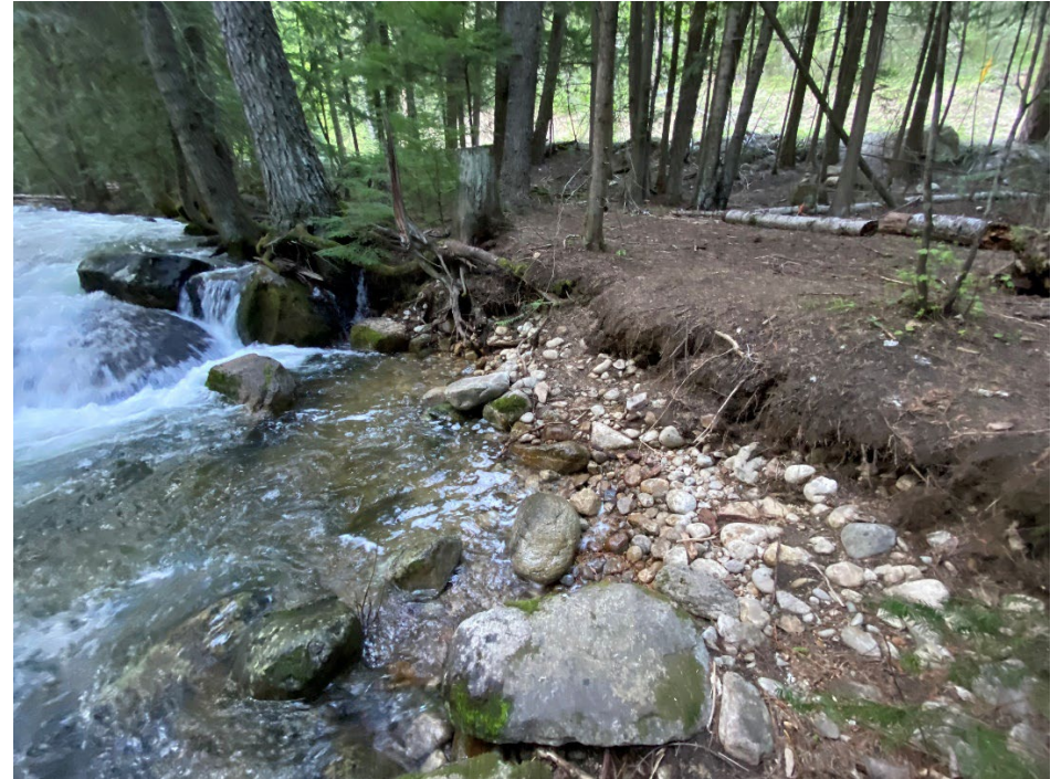
Bank erosion and trampled understory along the lower portion of Little Sand Creek.
