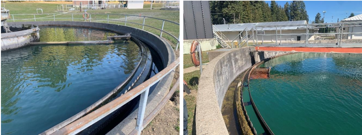
FIGURE 2-12: SECONDARY CLARIFIERS
