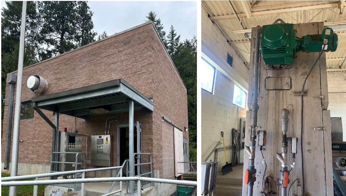
FIGURE 2-1: HEADWORKS BUILDING AND SCREEN
