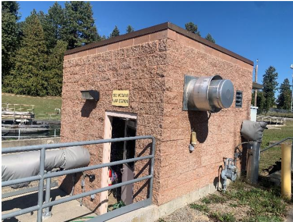
FIGURE 2-22: NON-POTABLE WATER PUMP STATION BUILDING
