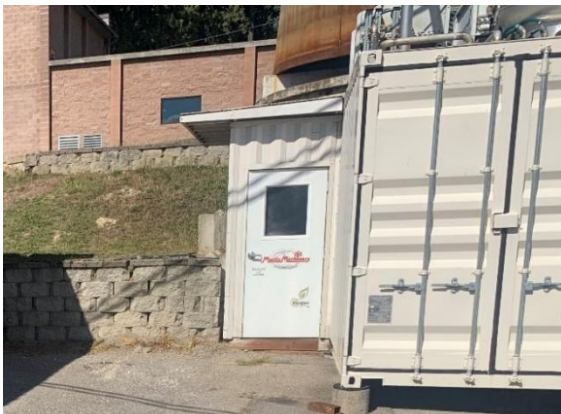
FIGURE 2-23: COMBINED HEAT AND POWER CONTAINER AND ENGINE
