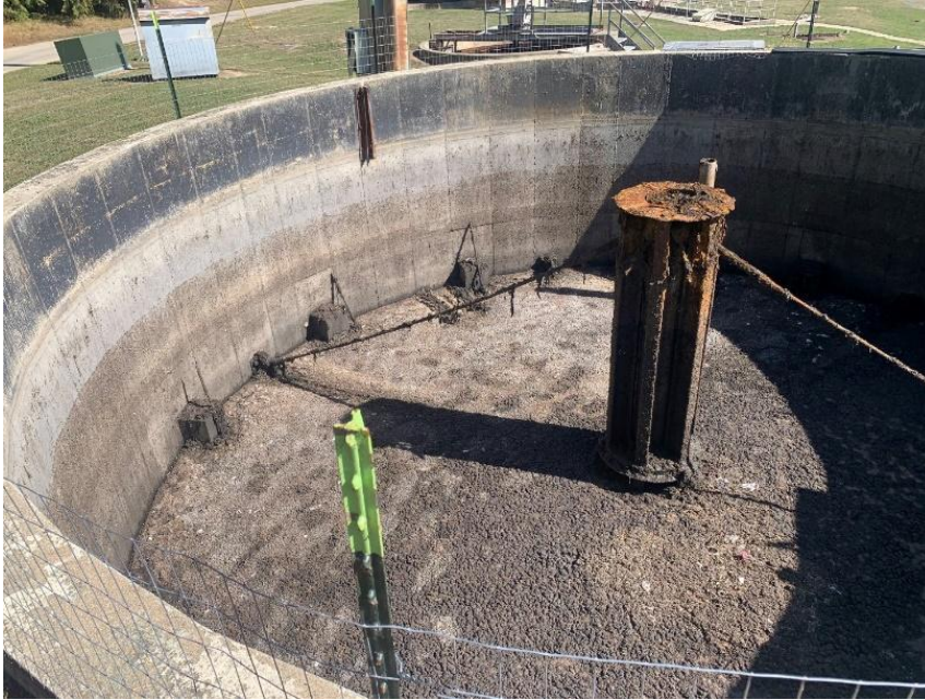
FIGURE 2-17: SLUDGE STORAGE TANK
