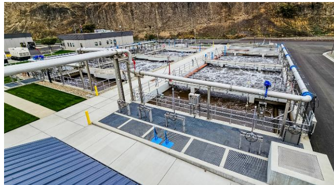
FIGURE 3-1: CONVENTIONAL ACTIVATED SLUDGE
