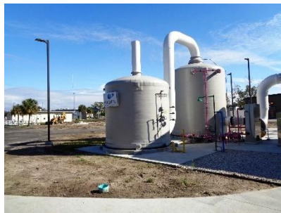
Biotrickling Filter
