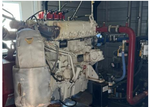
FIGURE 2-23: COMBINED HEAT AND POWER CONTAINER AND ENGINE
