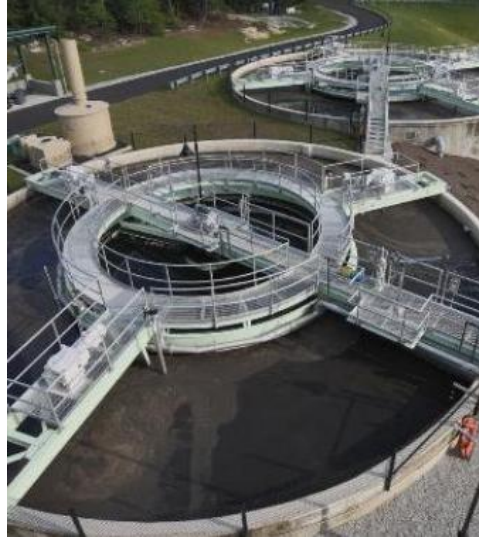
FIGURE 3-5: BALLASTED ACTIVATED SLUDGE
