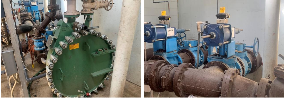
FIGURE 2-20: HEAT EXCHANGER AND SLUDGE MIXING LINES
