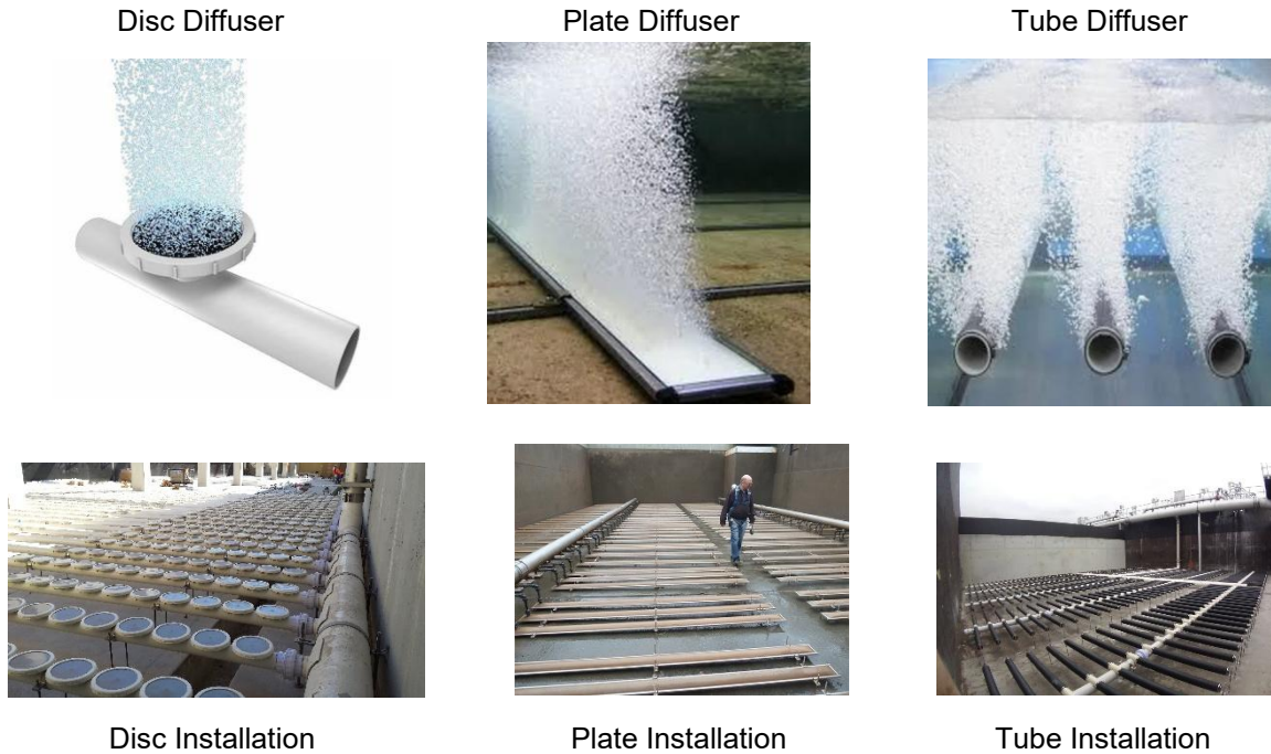
FIGURE 3-18: AERATION BASIN DIFFUSER ALTERNATIVES
