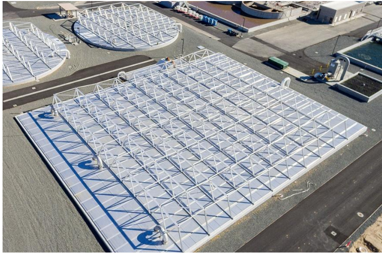
FIGURE 3-11: EQUALIZATION BASIN
