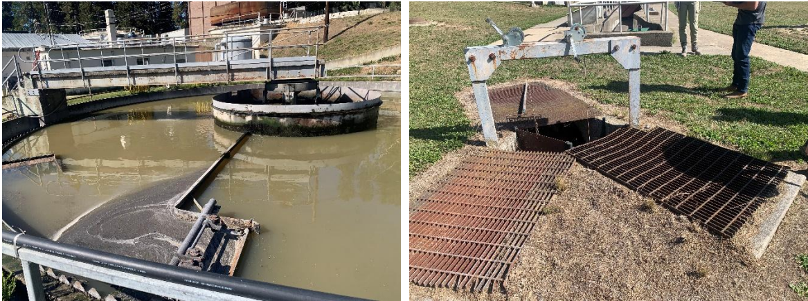
FIGURE 2-4: PRIMARY CLARIFIER AND FLOWS SPLIT
