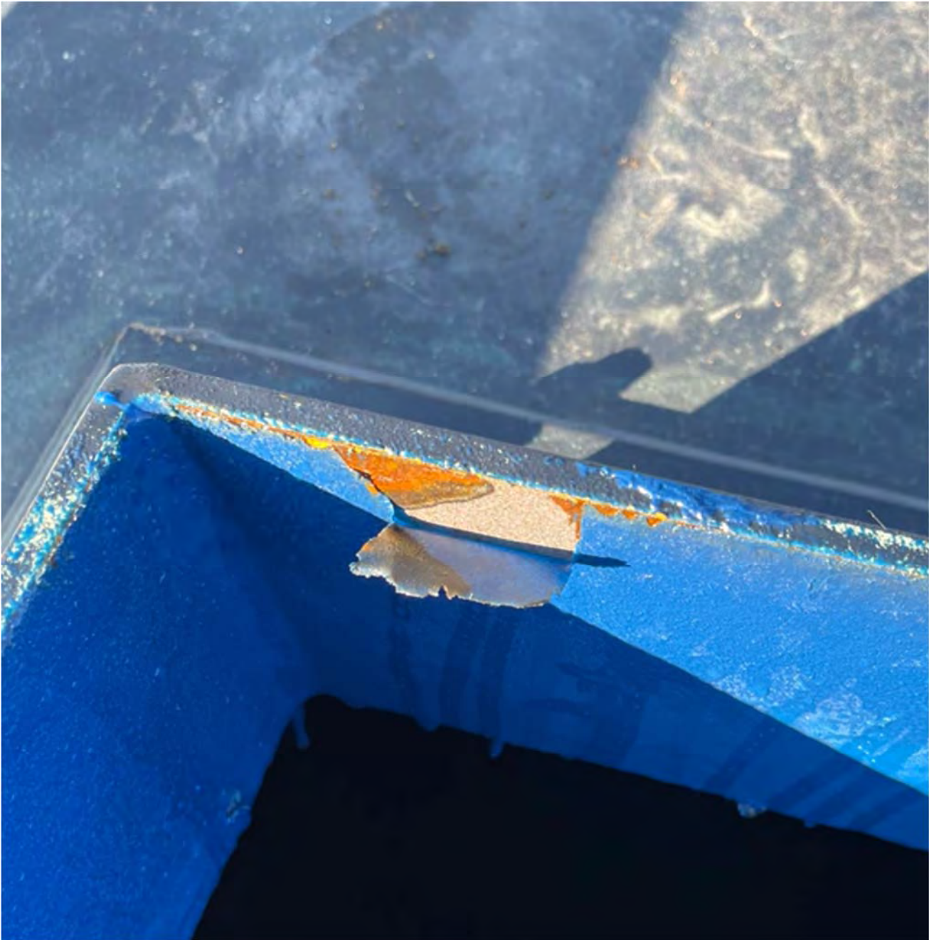
FIGURE 15 - PEELING LINER, UPPER HATCH RIM
