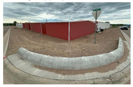
Currently, several inches of sediment deposition exist above the concrete foundation wall of the SMC shop, localized to the northwest building corner. Also, rilling and pronounced flow-line erosion are evident along the road shoulder ditches leaving the intersection in both directions along the building. Acute erosion is evident at the downspouts along the north side of the SMC building as well.
