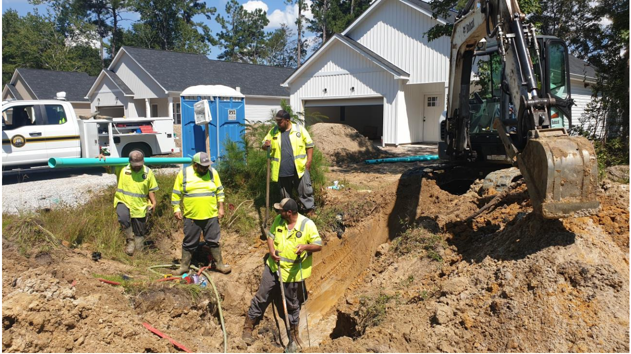
Installation of Gravity Sewer Taps
