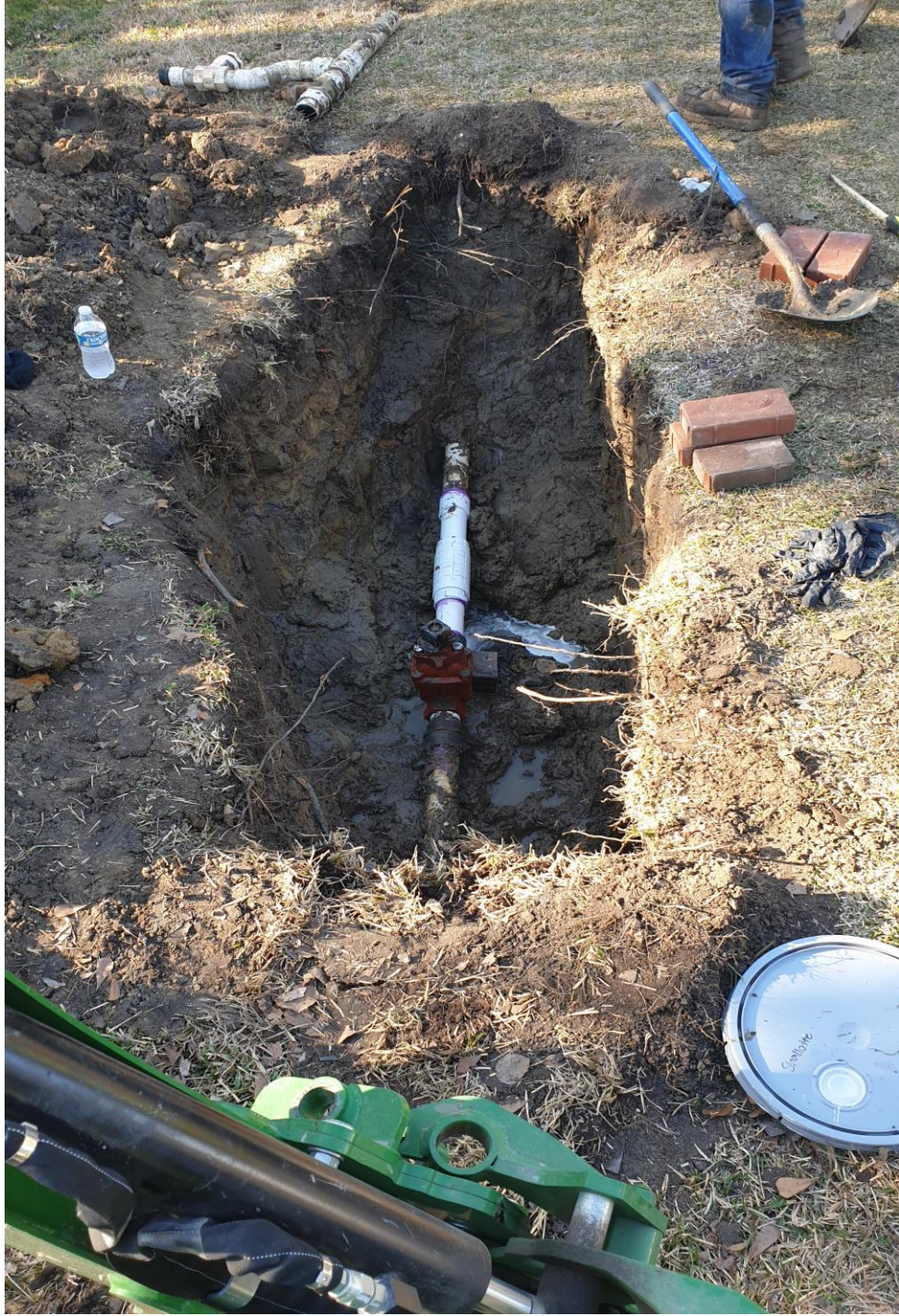
Replacement of original 40+ year old valve on Sand Trap
