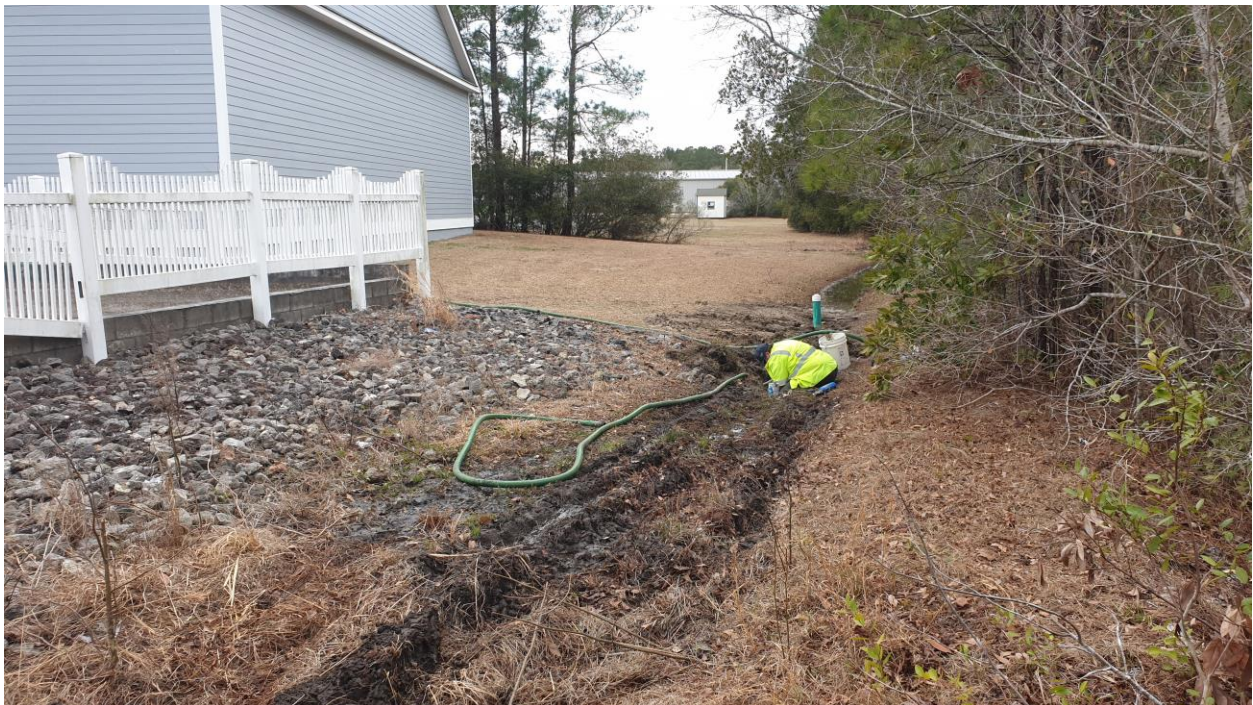
Gravity Sewer Repair
