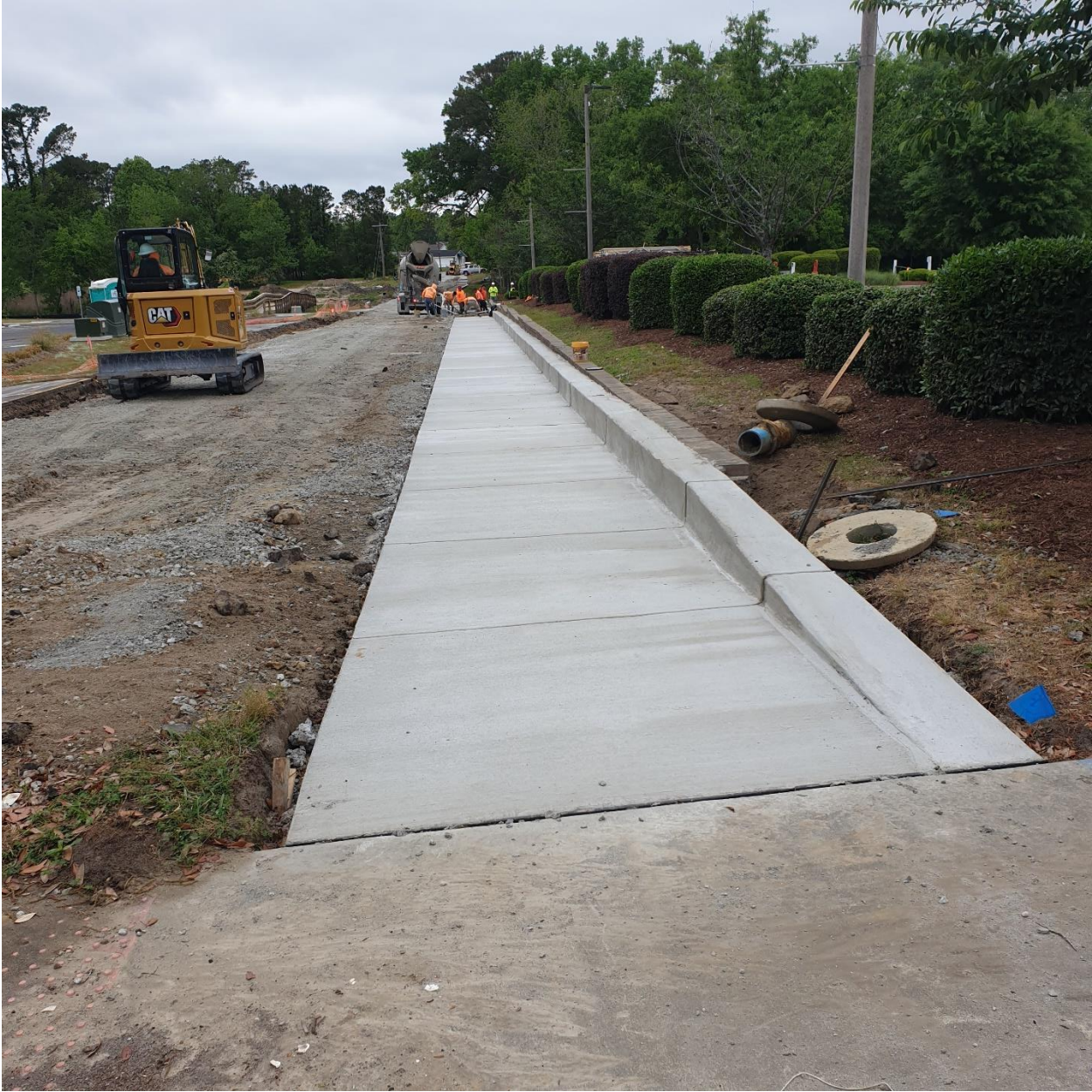
New sidewalk on Mulberry St.
