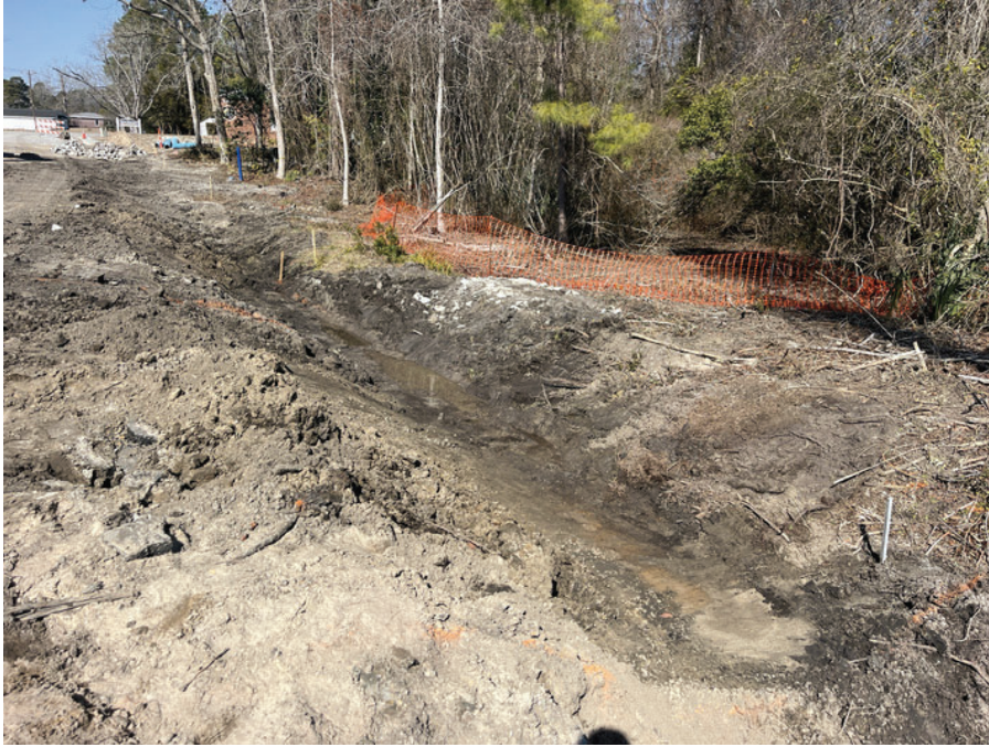
(P1) North end of Northwest retaining wall footing
