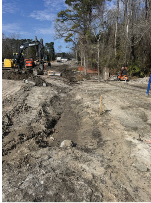
(P1) South end of wall
