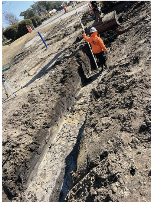
(P2) South end of Northwest retaining wall
