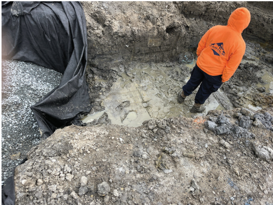
(P2) South end of Northwest retaining wall
