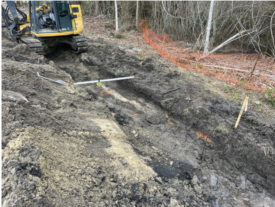
(P1) North end of Northwest retaining wall
