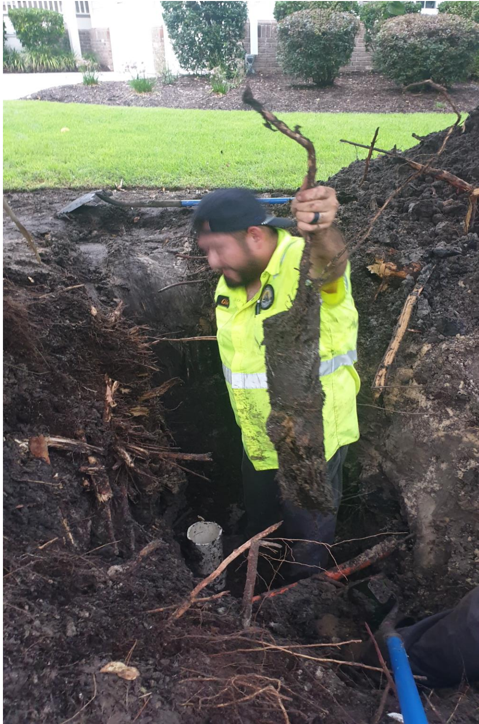
Root Removal From Gravity Sewer Service
