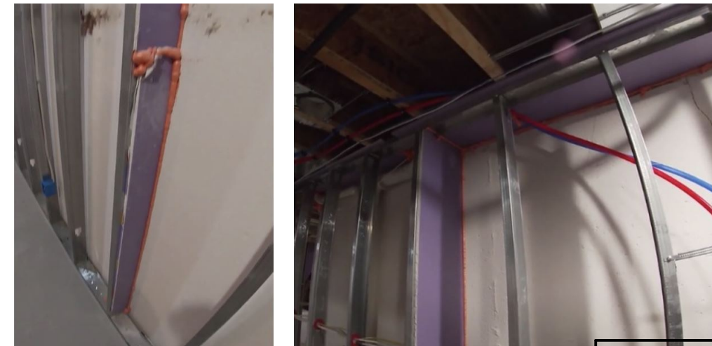
EXTERIOR WALL CORNER FRAMING
