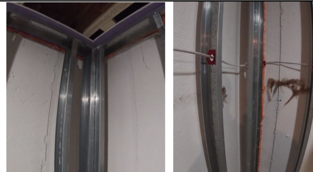
EXTERIOR WALL FIREBLOCKING
