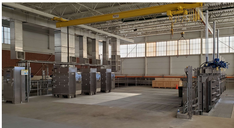
New Trojan UV Disinfection System – MMSD.
