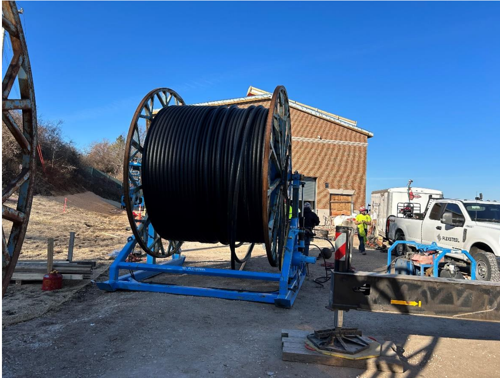
Intake chemical feed line spool set up for pull.
