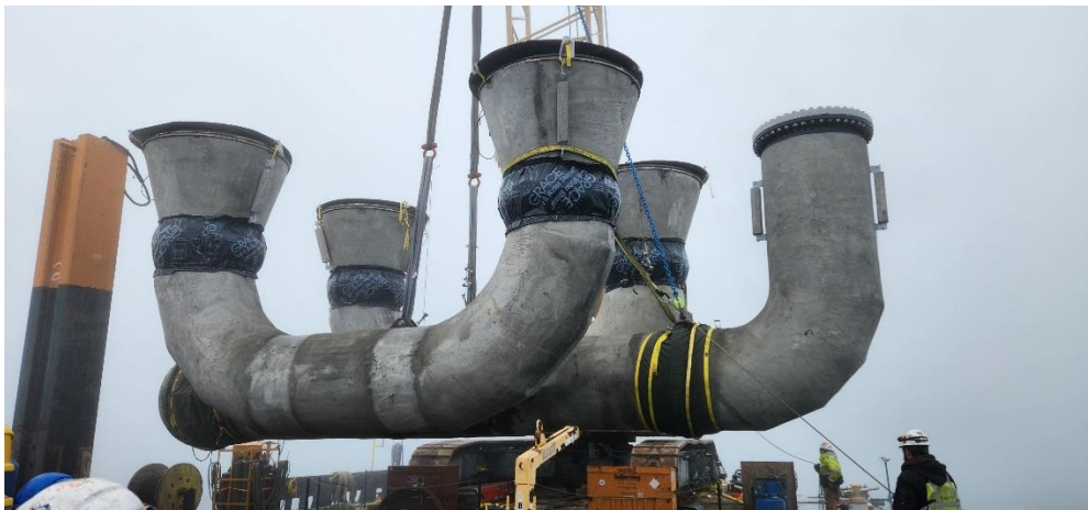
Intake structure lifted off crane barge.
