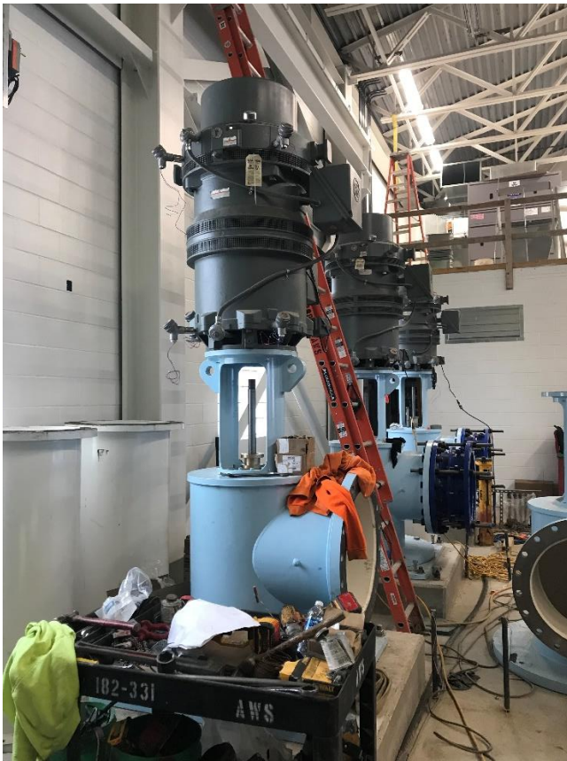
Vertical turbine pump and motor installation.
