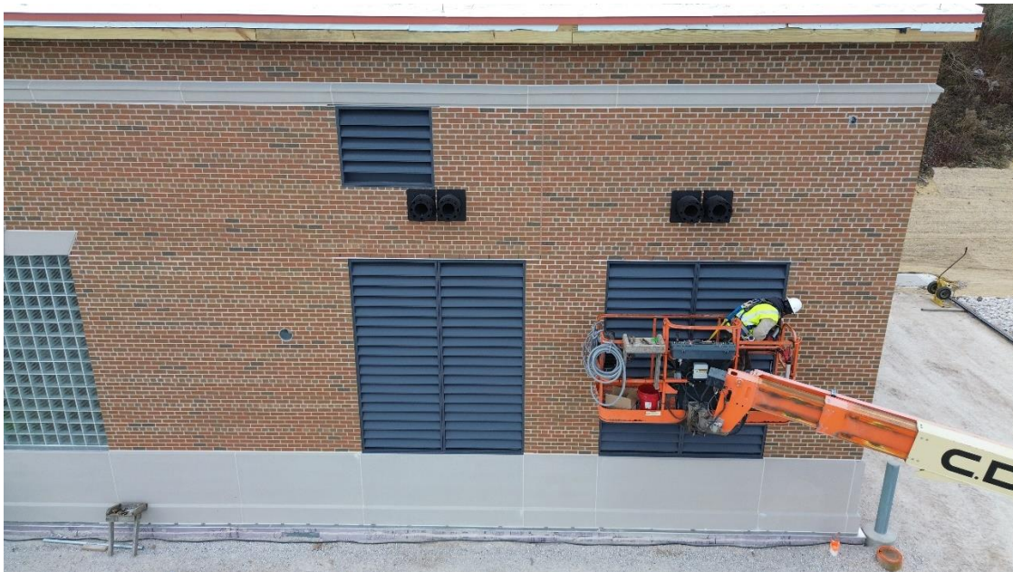
Exterior masonry joint caulking.
