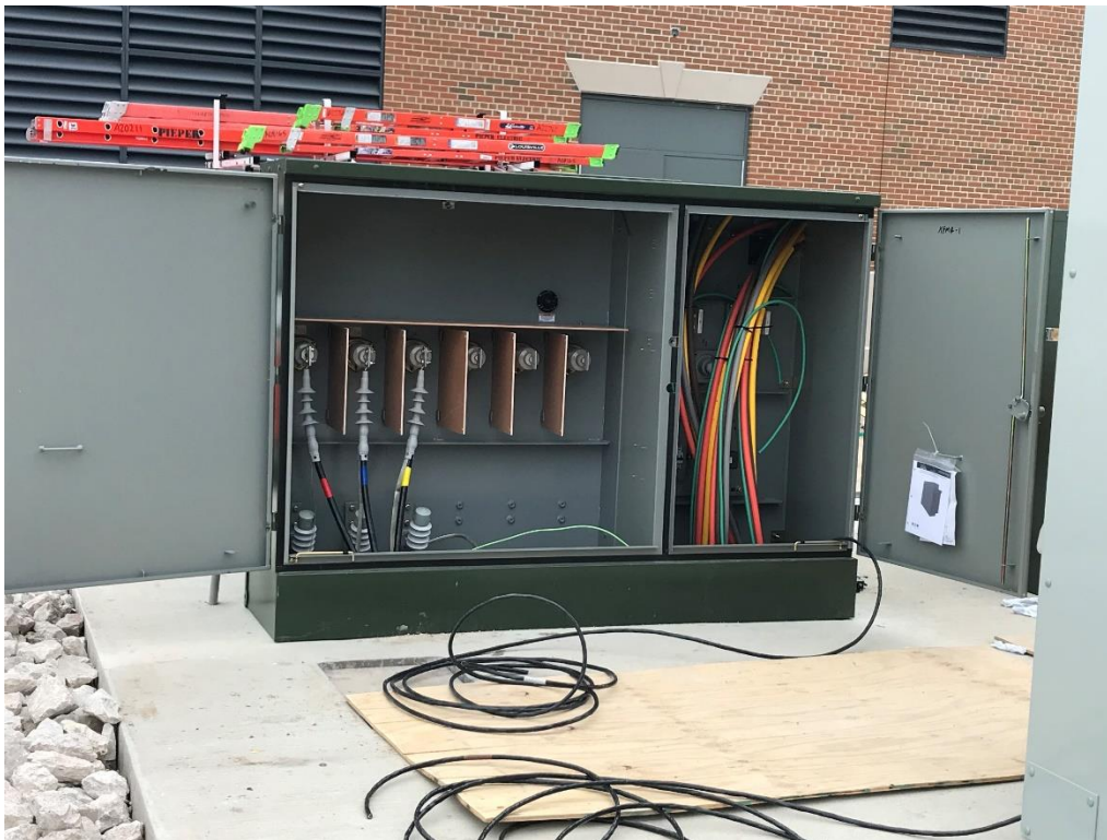
Electrical cable terminations at transformer.
