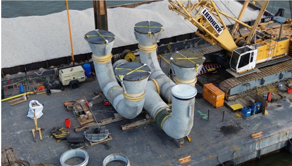
Intake structure assembled on crane barge.
