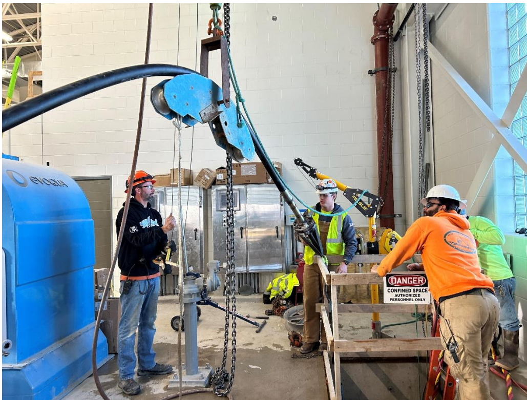
Chemical feed line pulling head positioned for pull.
