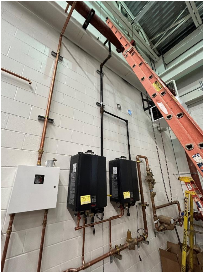
Water and gas pipe connections at water heaters.
