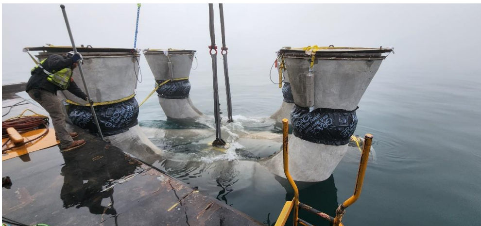
Intake structure submerged into position.
