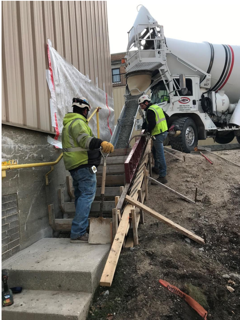
Concrete stair placement adjacent to garage.
