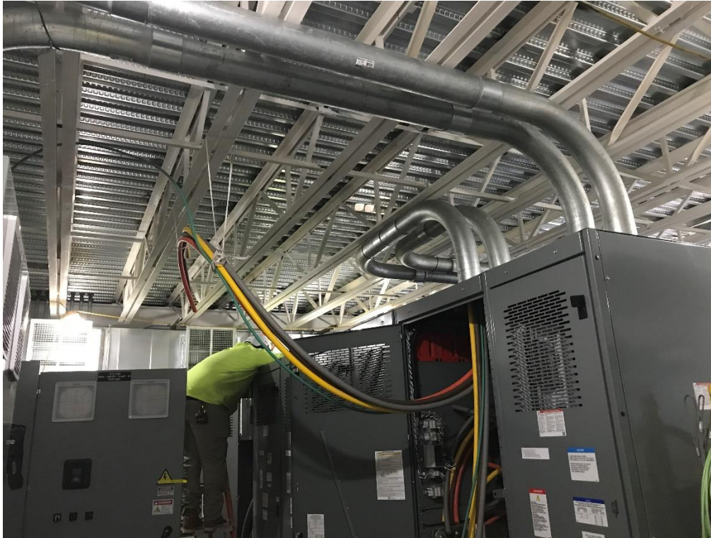
Electrical gear assembly and conduit installation.
