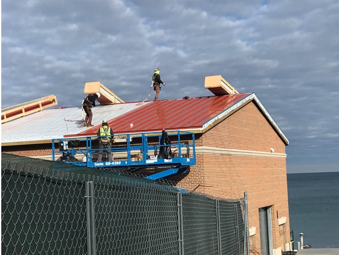
Standing seam metal roof installation activities.
