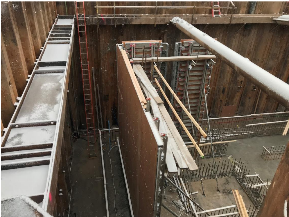
Pump station wet well wall form erection.
