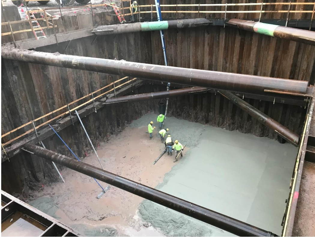
CDS places mud slab at bottom of pump station excavation.
