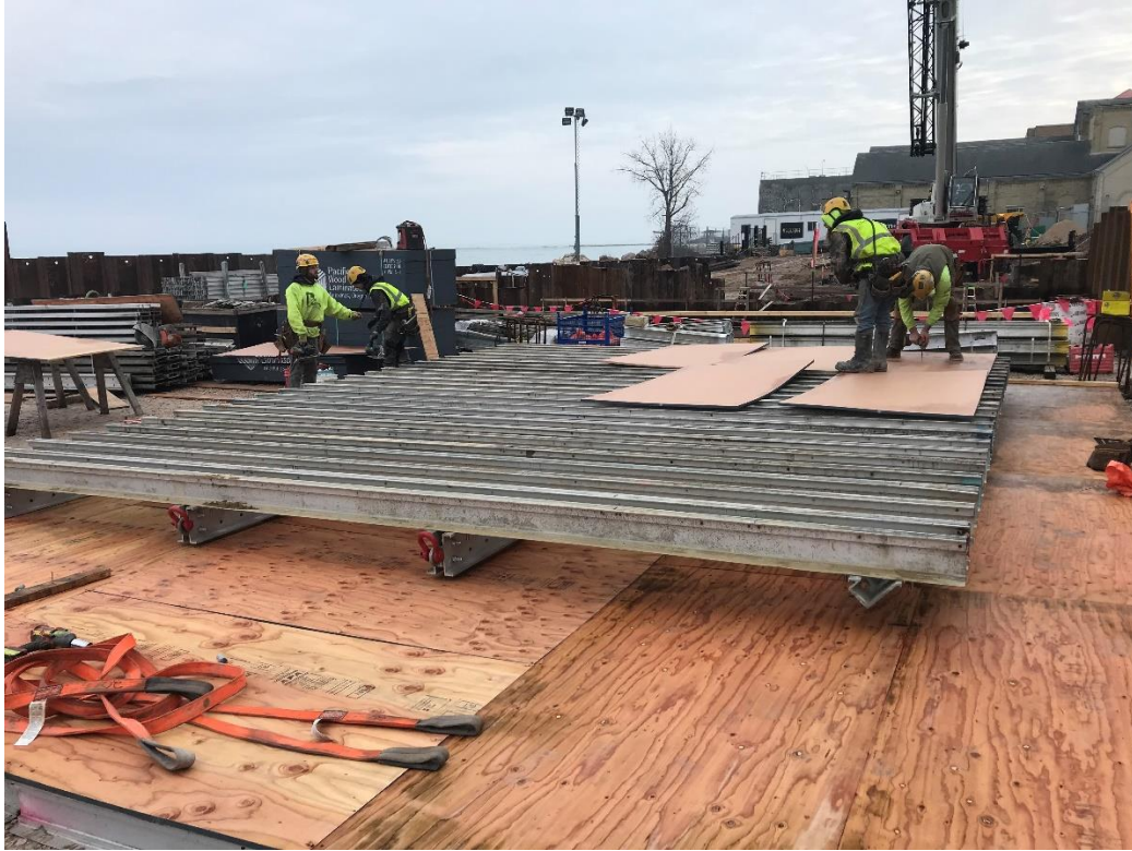
CDS assembles wet well wall form panels.
