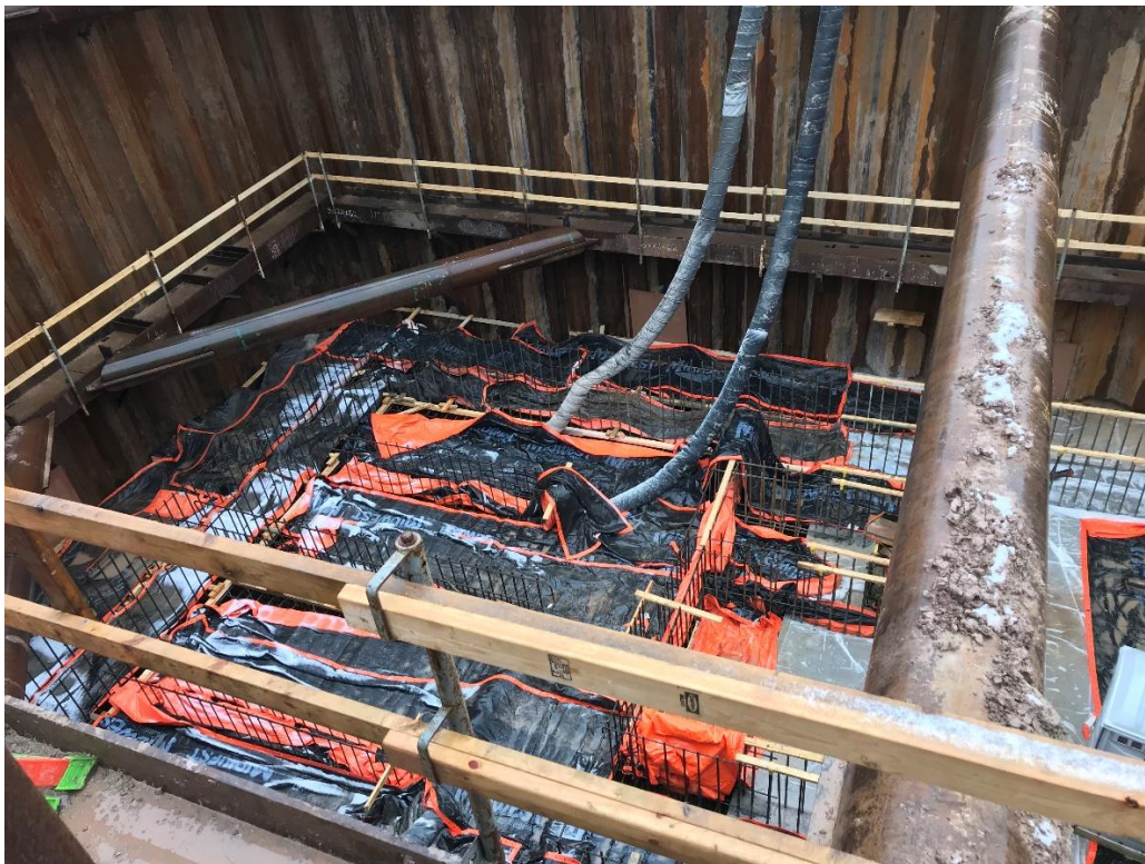
Pump station base slab area heated prior to concrete placement.
