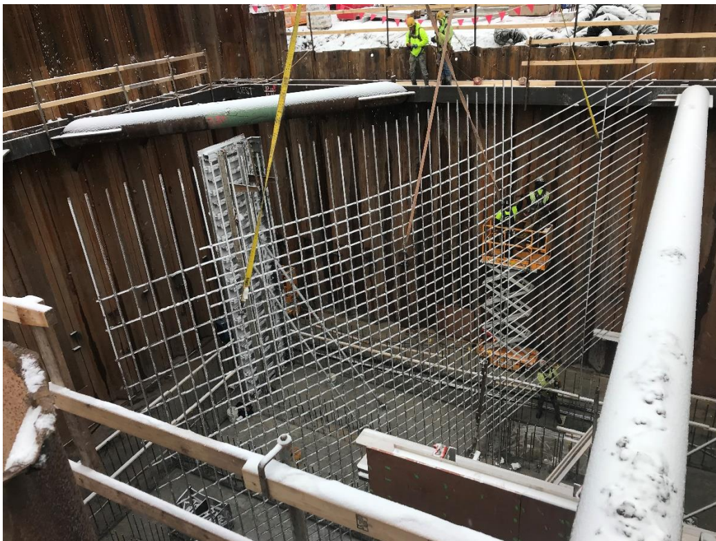
Wisconsin Rebar sets wet well rebar wall mat.
