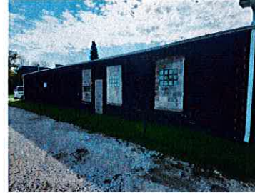
EXISTING ALLEY ELEVATION - BUILDING #1
