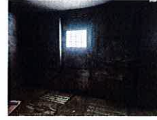
EXISTING INTERIOR VIEW #1
