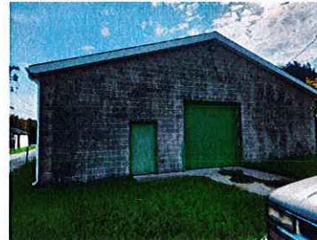
EXISTING BUILDING #2 - REAR ELEVATION
