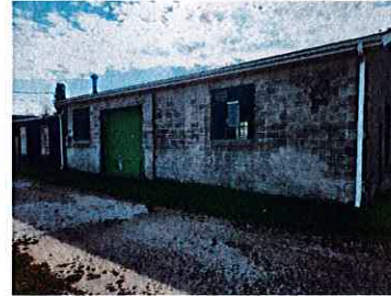
EXISTING ALLEY ELEVATION - BUILDING #2
