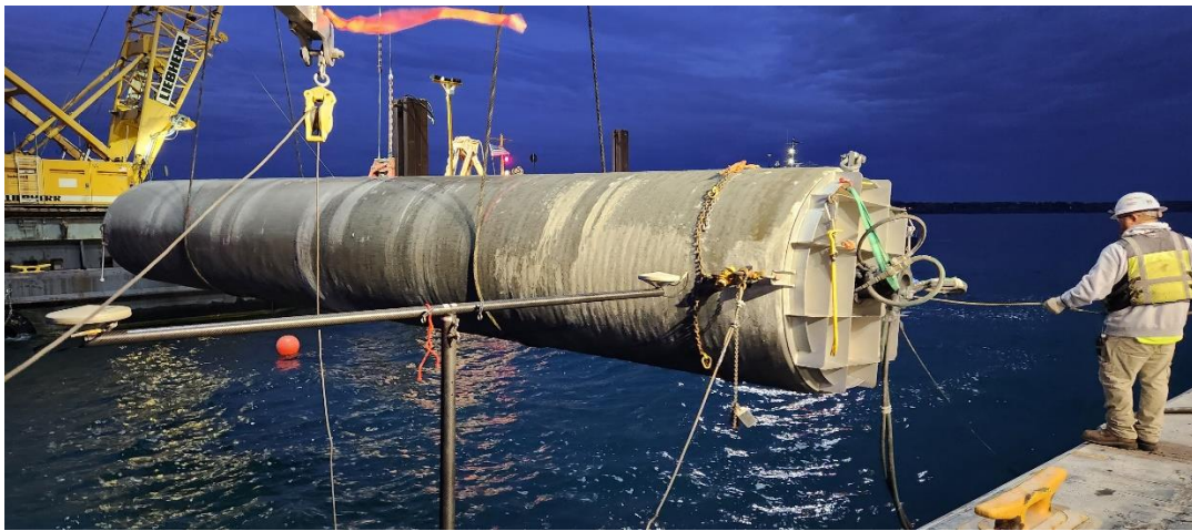
Kokosing installs main line intake pipe.
