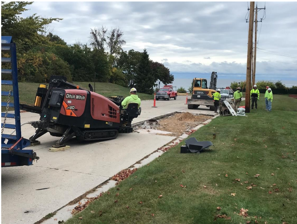
3" sanitary pipe installed with horizontal directional drill at Vollrath Blvd.
