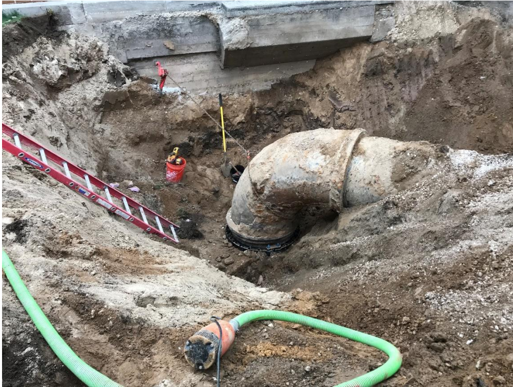
Existing 36" RW pipe exposed at tie-in location.
