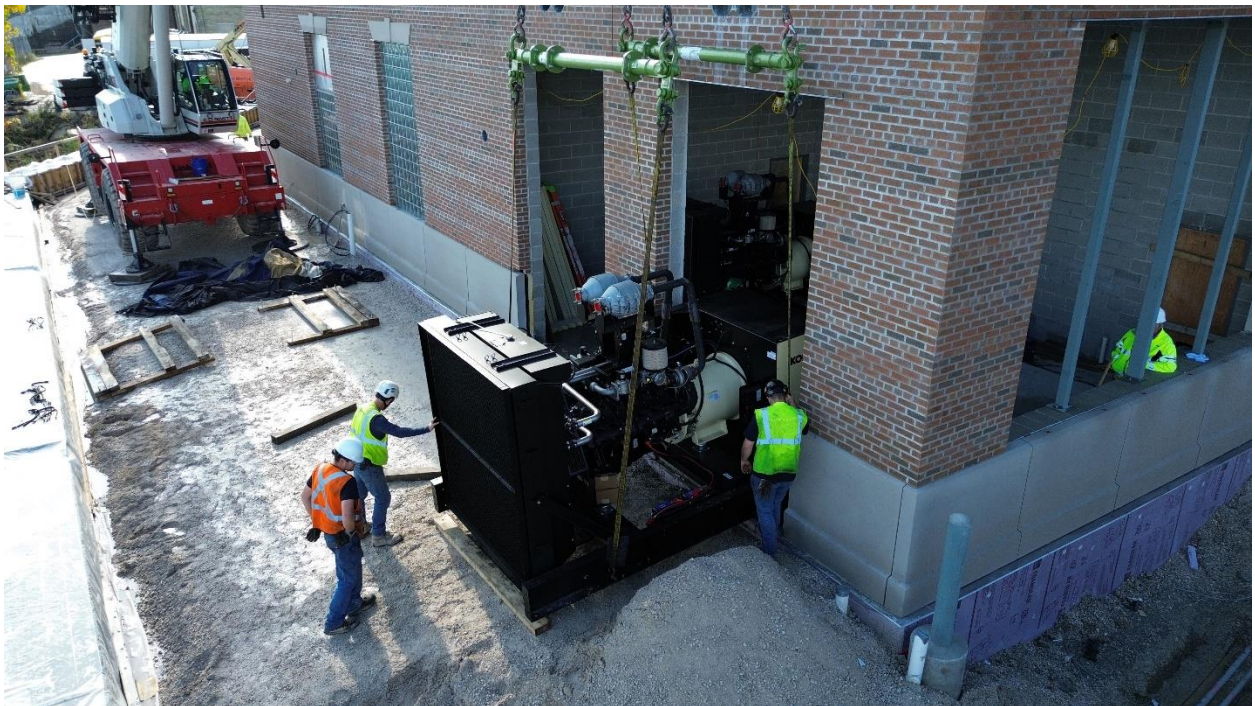
Kohler generator installed through louver opening at pump station generator room.
