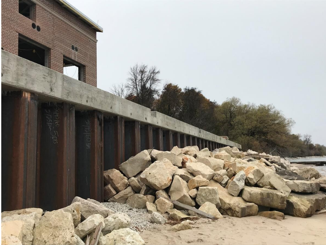
Revetment sheet pile concrete cap.
