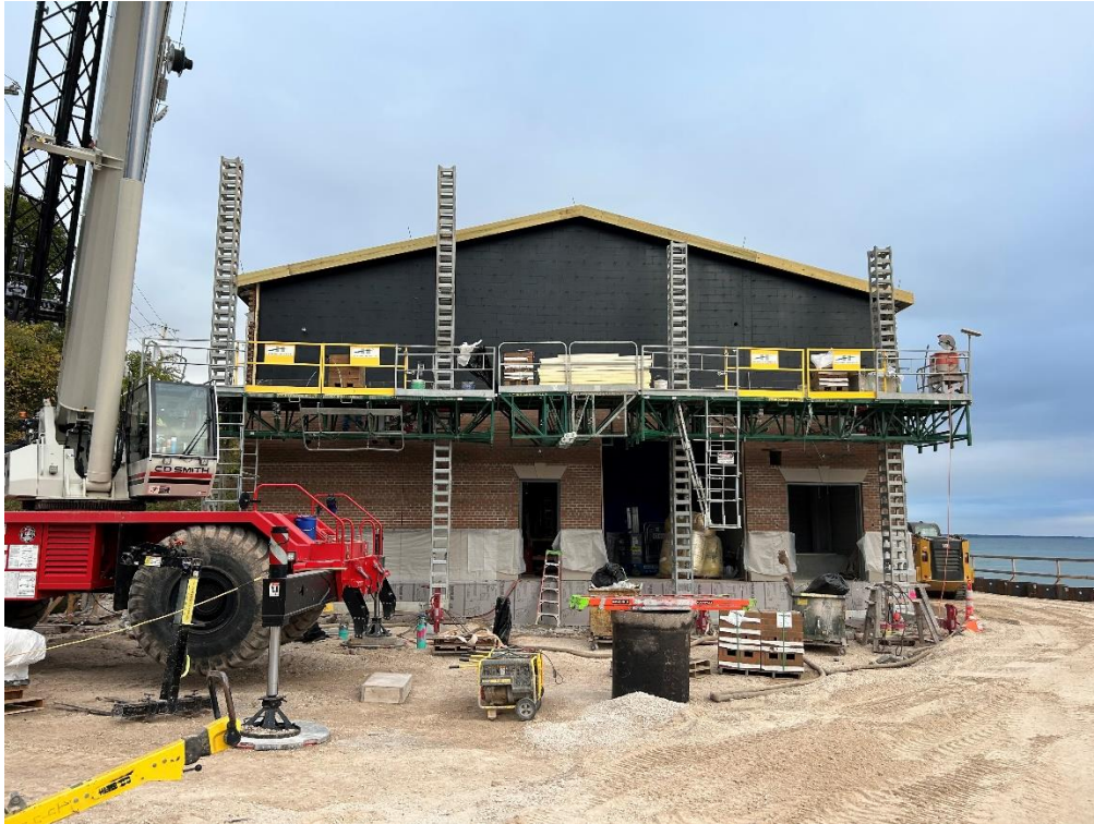
Face brick installation at south pump station elevation.
